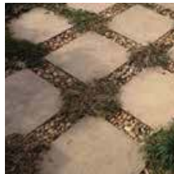
Pavers in gravel bed
