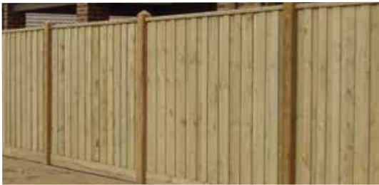
Capped timber palings with exposed post
